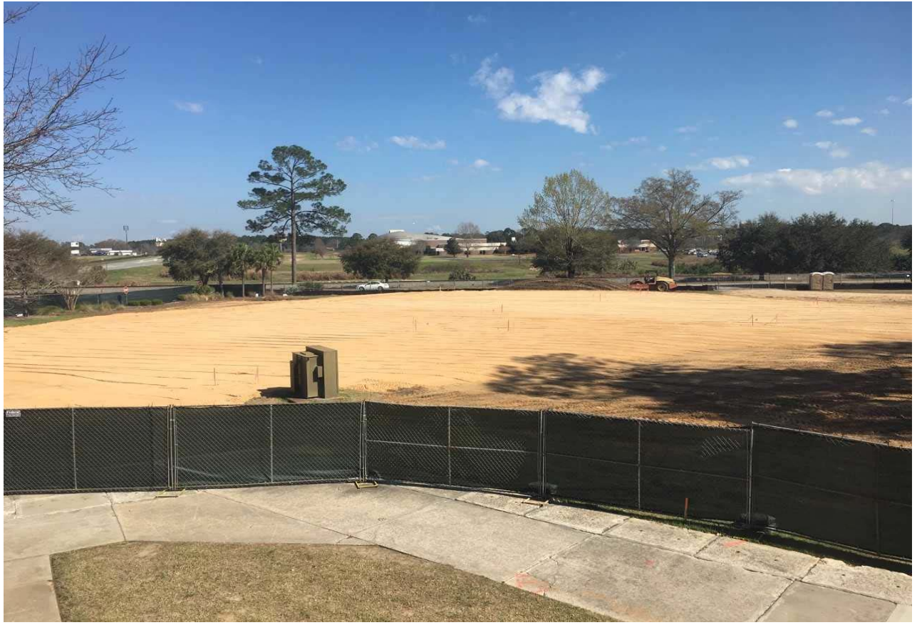
Update 2/22/19 - Grading complete for the new Fine Arts building
