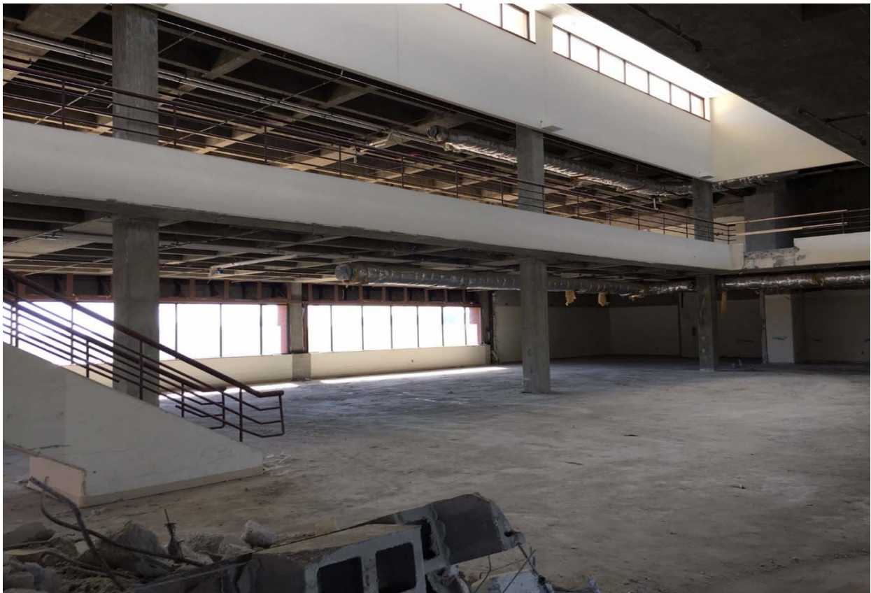
Update 1-22-2019 - Selective demolition of the Carlton Center interior continues
