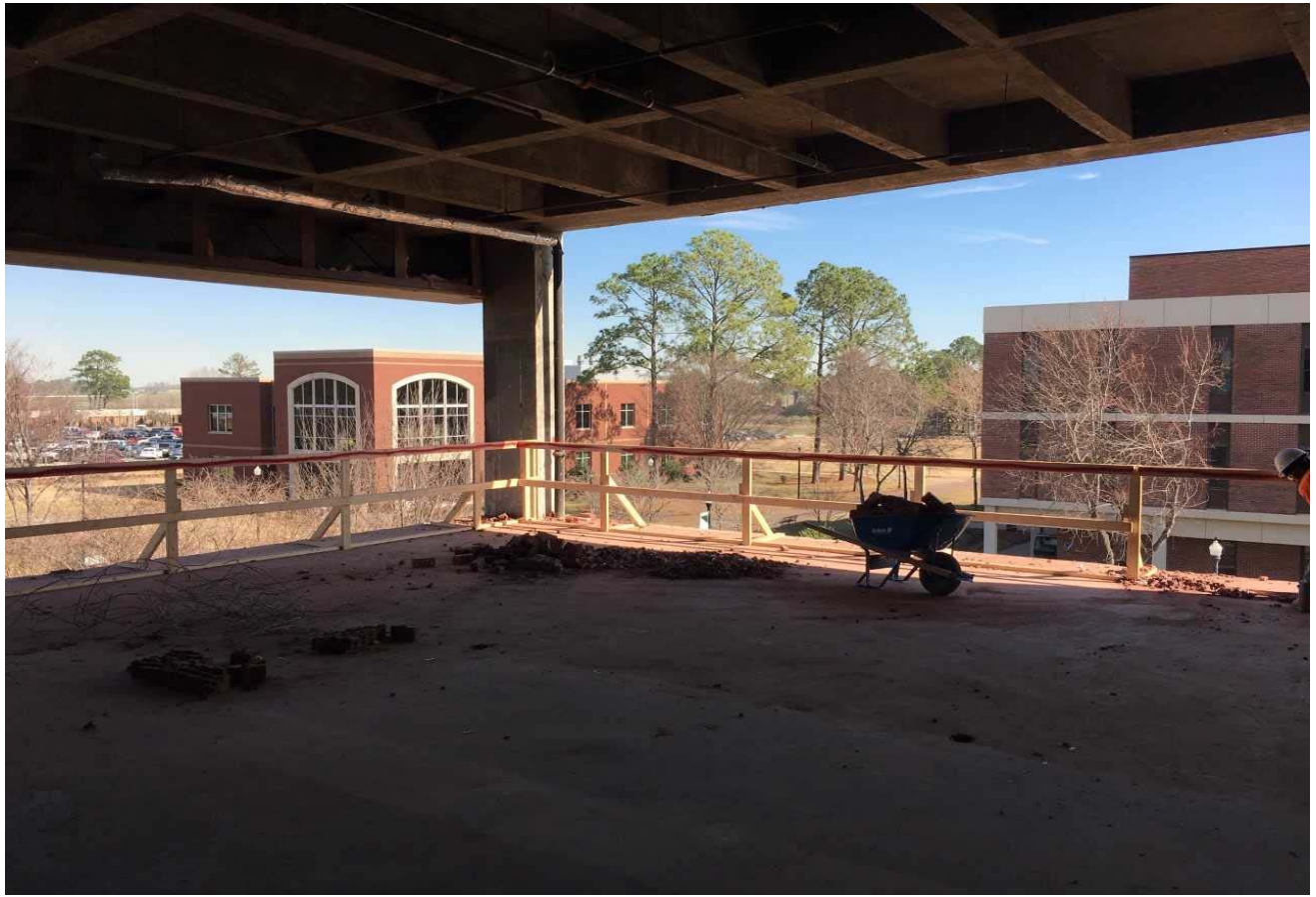
Update 2-12-2019 - Demolition continues - 3rd floor looking northeast
