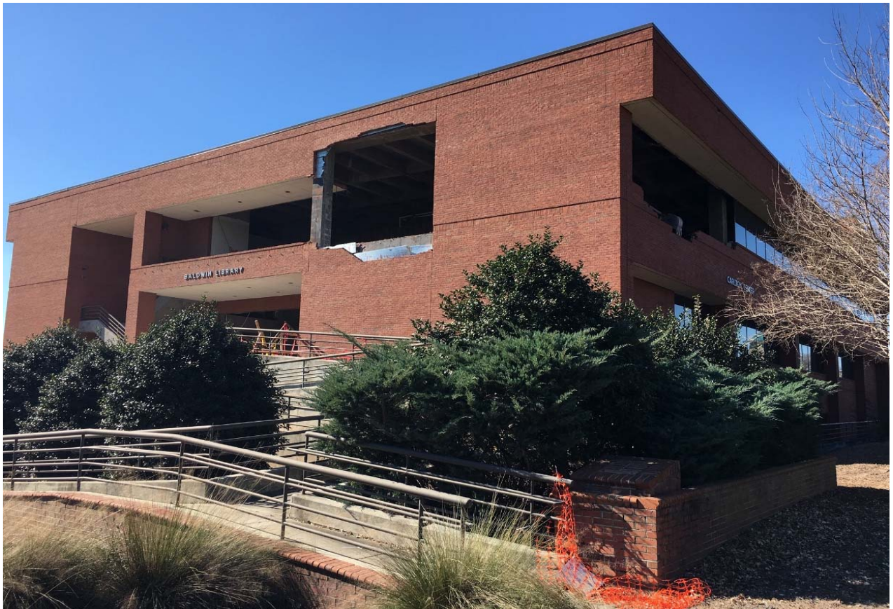
Update 1-28-2019 - Selective demolition of the Carlton Center continues
